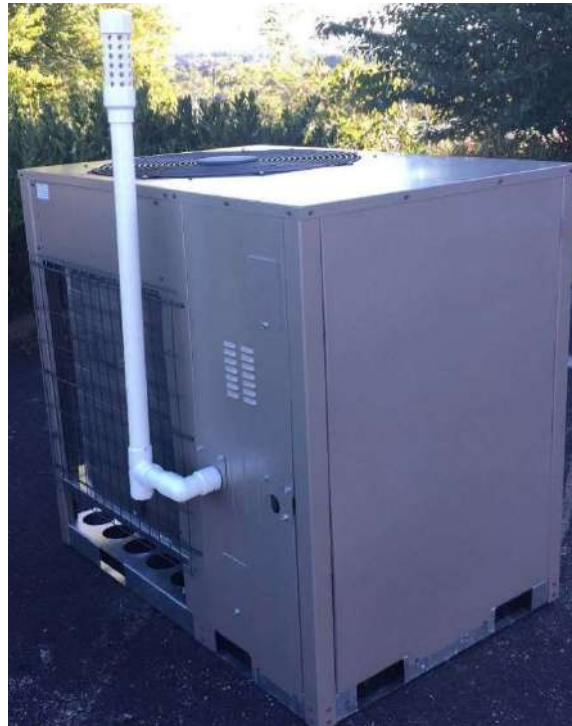
Figure 6. An 80,000 BTU/hr gas absorption heat pump using ammonia-water as working fluids at a field test site (Courtesy: SMTI, USA).
