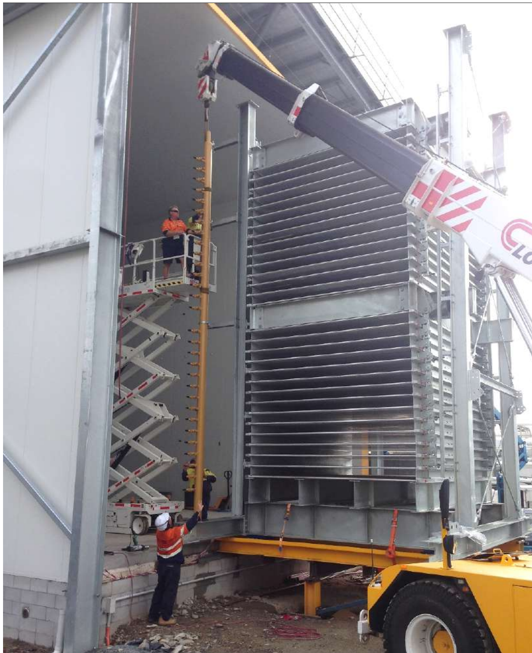
Figure 9. Large-scale automatic plate freezer for 60 lb. meat cartons during installation.
