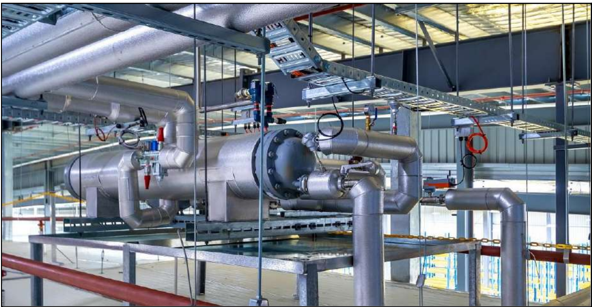
Figure 12. Shell-and-tube DX \text{NH}_3 heat exchanger for chilling a mixture of propylene glycol and water.
