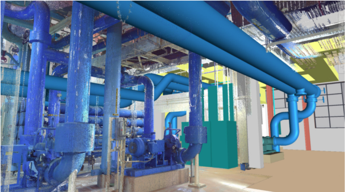
Figure 6: Isometric view of 3D scan combined with the design model.
