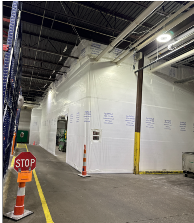
Figure 3: An example of temporary plastic walls.
