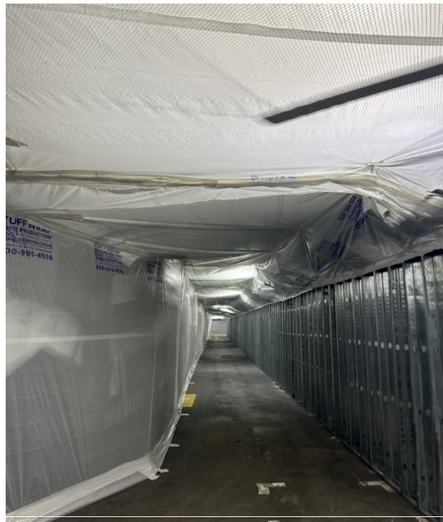
Figure 2: Example temporary tunnel with metal stud wall and plastic tunnel.
